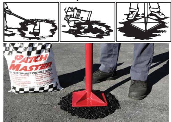
Figure 1. Cold-patch method for pothole repair [11].
