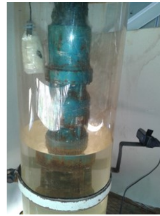
Figure 3. Submersible pump and connection of the camera
