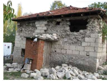
Figure 4. Typical damage pattern in Çameli earthquake
