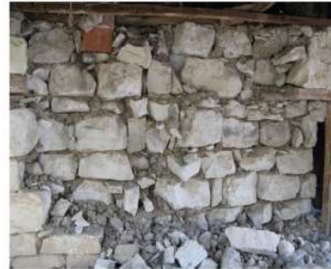
Figure 5. Unconnected outer and inner wiches
